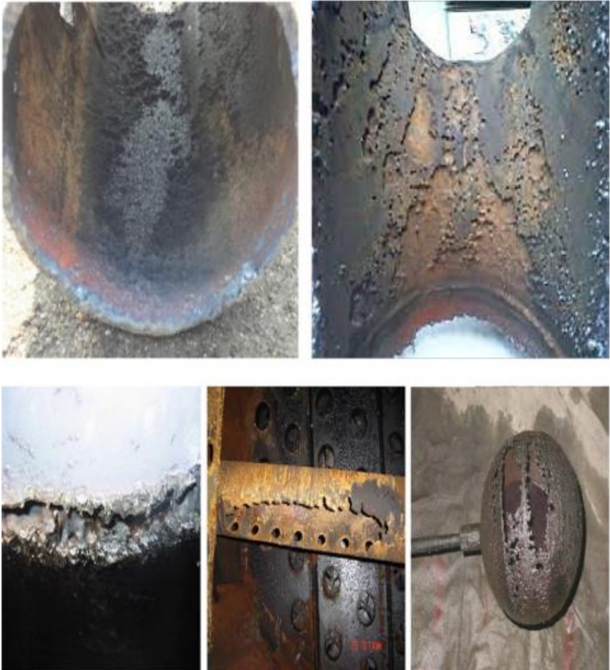
Figure 2: Resultant effect of naphthenic acid being corroded (NA),. (Source: reference [3])
