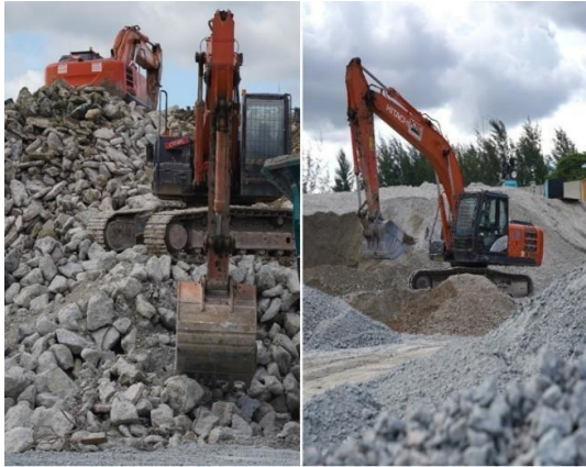
Fig. 1: Collection of demolished concrete
