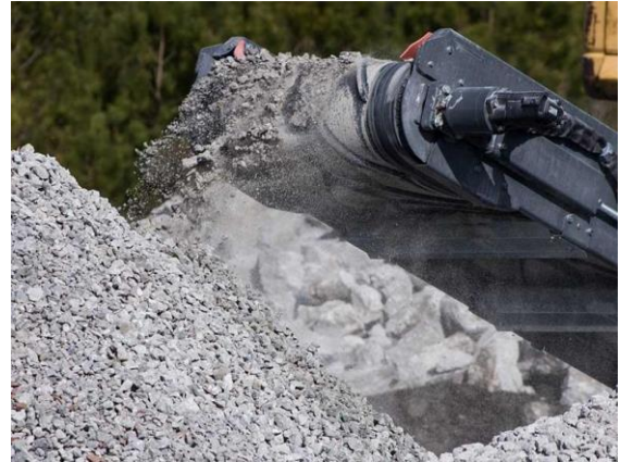
Fig. 2: Recycling of demolished concrete
