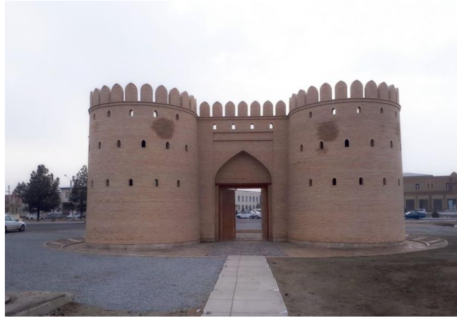
Figure 6. Hazrati-Imam gate current status view
